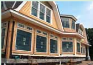
Insulated Concrete Forms (ICF) Home Mason's Island M.H. Lyons
